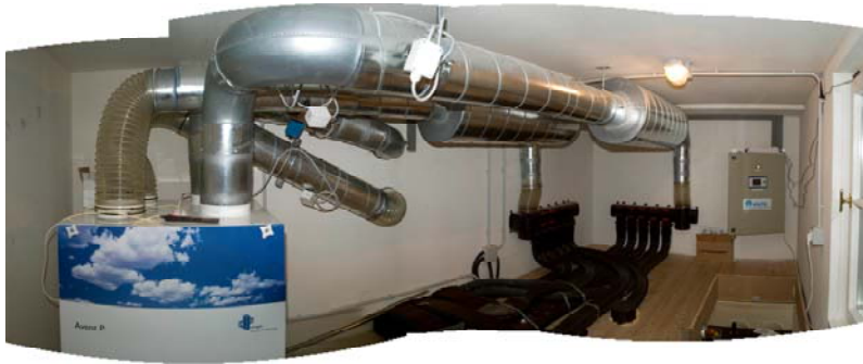
Figure 7. Technical installation (e.g. the ventilation system) were positioned in a new “plant room” above the kitchen, taking advantage of the amply height of the rooms
