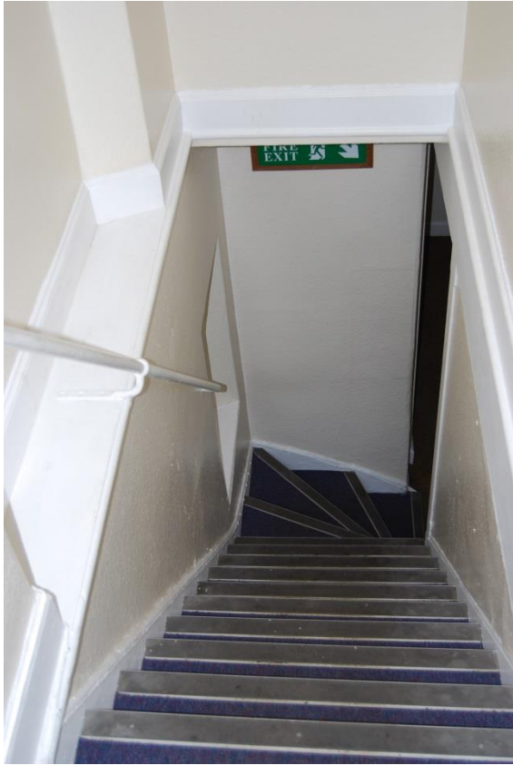
Figure 23: Carpeted, narrow stairway providing access to first floor.
