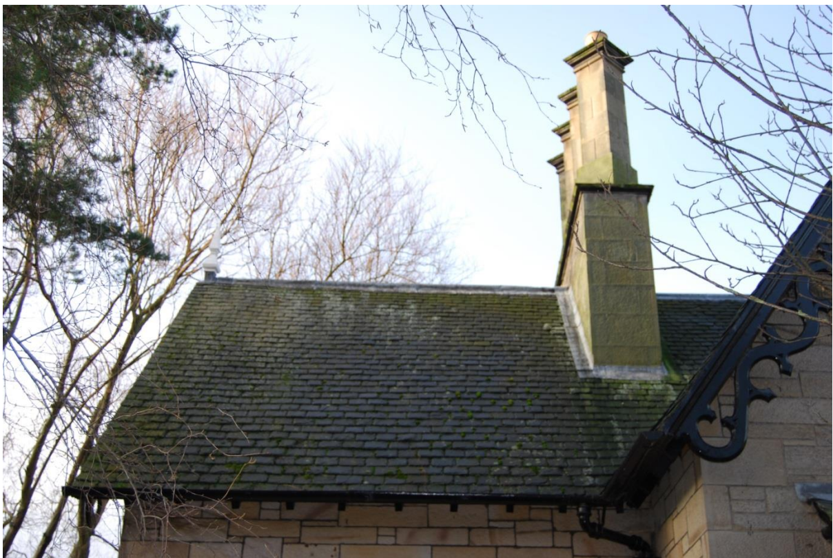
Figure 4: West elevation of the roof
