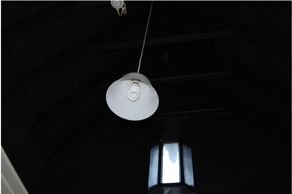
Figure 13: Exposed rafters in entrance lobby, uninsulated and painted black.
