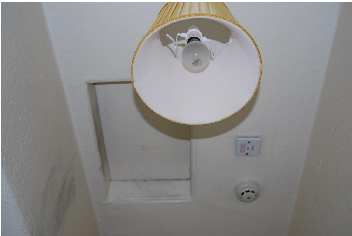
Figure 26: Small hatch above stairs offering access to the northern attic space.
