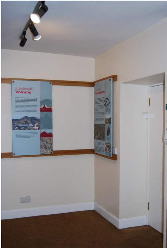
Figure 15: Carpeted, uninsulated floors.
