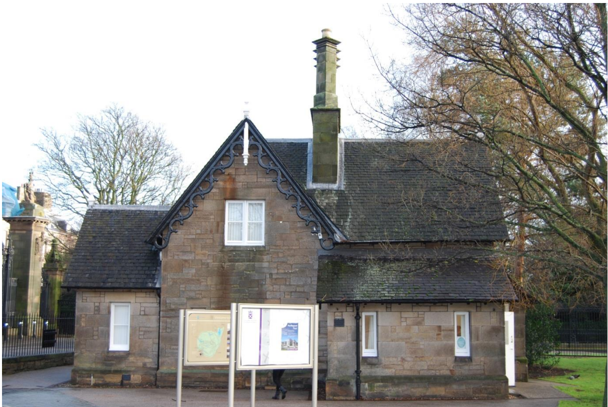
Figure 2: West elevation of the lodge showing the overall external condition
