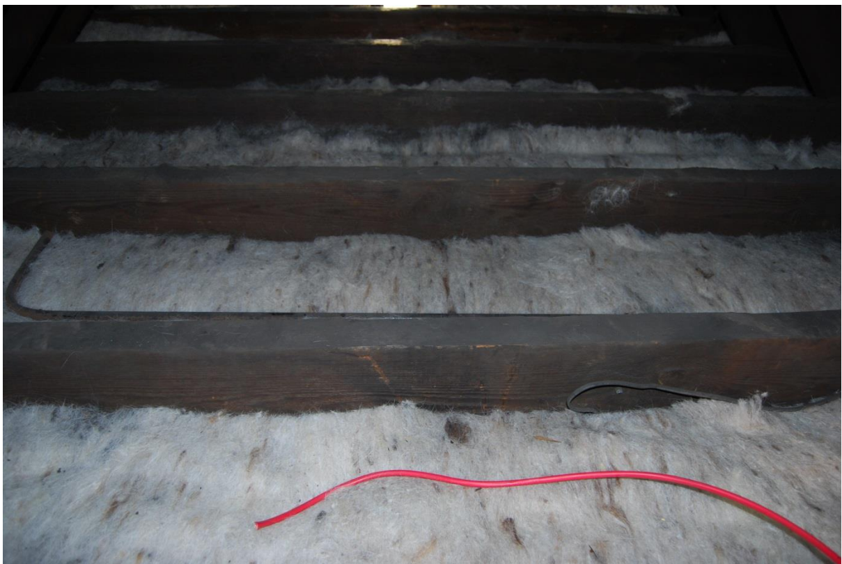
Figure 30: Sheep's wool insulation in between joists.
