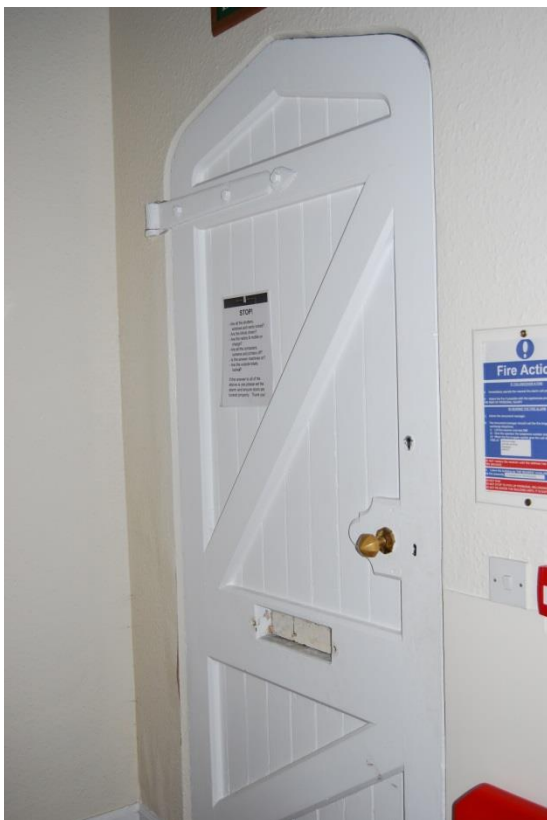
Figure 12: Timber ledge and braced external door fitted with no draught-proofing.
