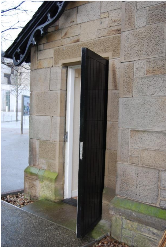
Figure 11: External timber panel door to exhibition space, usually left open.
