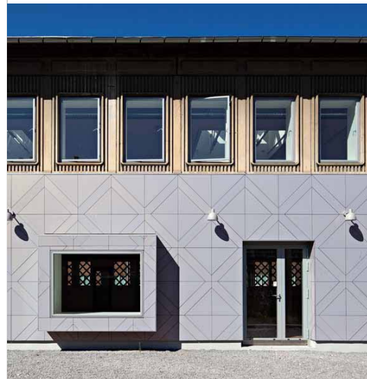
Façade facing garden - After renovation
