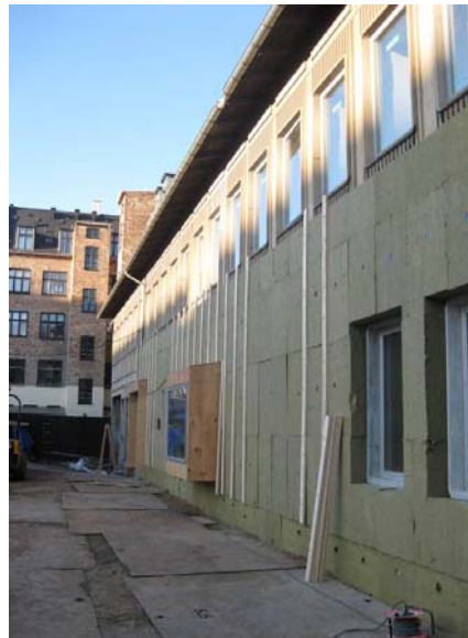
The ground floor of the back façade was insulated from the outside.
