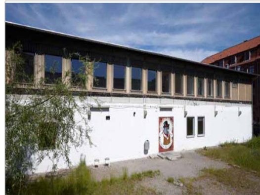
Façade facing garden - Before renovation
