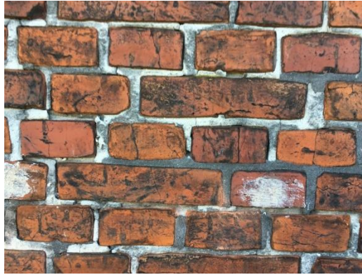
Figure 41: Face brickwork from RIBuild case study building Meinungsgade, Denmark.
